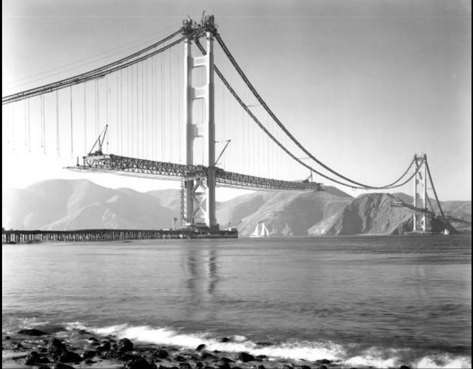
Golden Gate Bridge construction 1937
